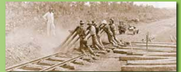
Putting in new siding for the farm, the first break in the line for 16 years, 1912 Federal Parliamentary Party Visit 1912. PH100/0069
